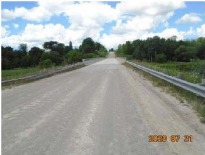
Images of Bridge in Excel Condition 10 th Line Bridge
