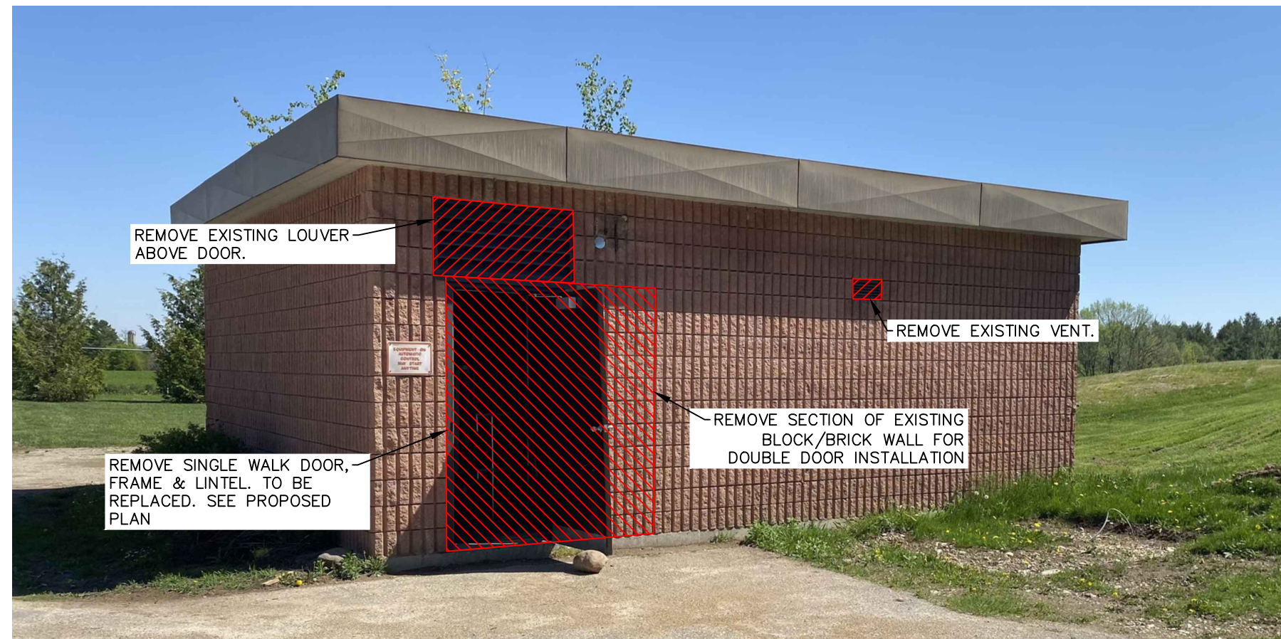
NORTH ELEVATION OF EXISTING FILTER BUILDING N.T.S.
